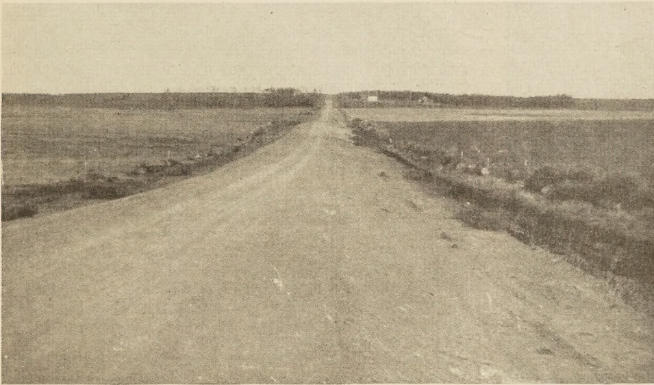
Tumbleweeds Caught Along Fence Lines May Cause Snowdrifts Across the Roadway During Winter Months.
